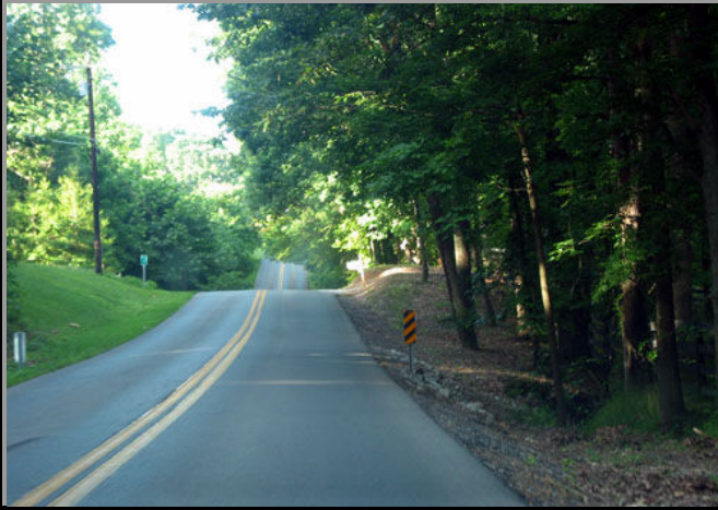
Figure 1.1, Difficult Vertical Alignment
