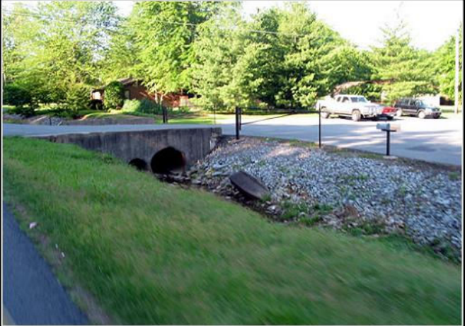
Figure 1.2, Deep Ditch at Road Edge
